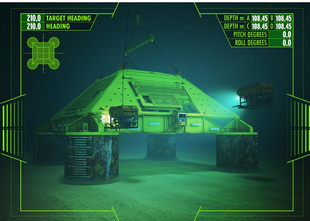
Ashtead Technology's dual independent DMS systems monitored and analysed parameters such as structure deflection, heading, pitch, roll and suction can differential pressures in real-time. This method of real-time monitoring is vital during the placement of suction can-based subsea structures as it ensures any potential issues can be acted upon immediately, reducing the risk of structural damage.
